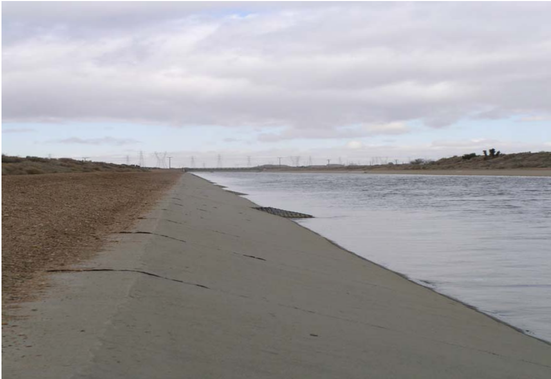
Figure 7-25. Drop Inlets Along the California Aqueduct in Hesperia
