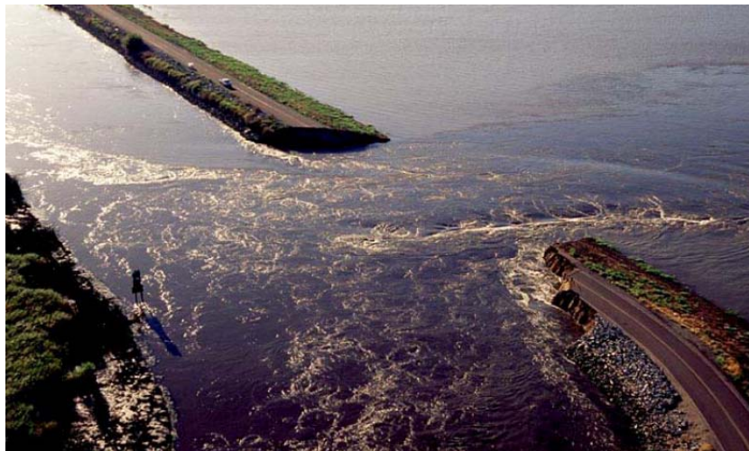
Figure 6-2. Levee Break on Upper Jones Tract
