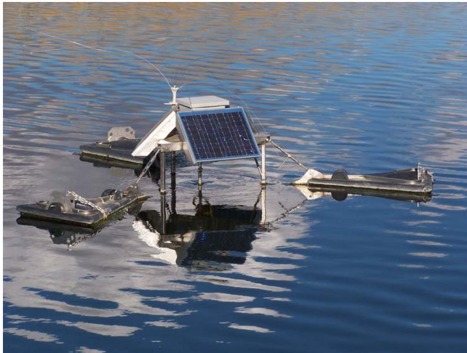
Figure 7-22. Installation of SolarBee® at Polonio Pass Pumping Plant Forebay
